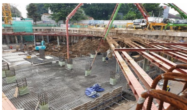
Gambar 1. Rangka strutting (Sumber : PT. Yodya Karya Persero, 2021)
