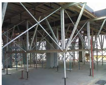
Gambar 5. Bekisting aluma system
