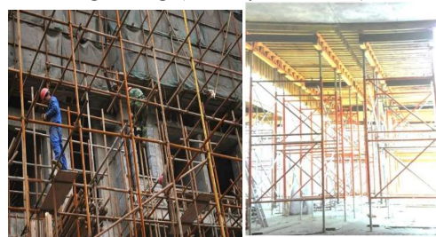
Gambar 1. Bekisting scaffolding ( www.pengadaan.web.id/2020 )
