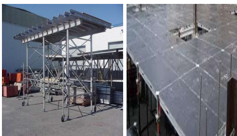
Gambar 2. Bekisting Aluma System (Hadi, 2019)
