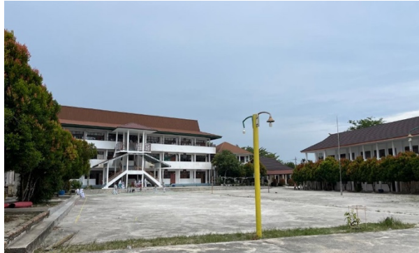
Gambar 1. Gedung MTs Hidayatul Ma’arifiah
