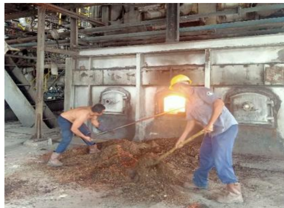
Figure 2. The Addition of Boiler Fuel
