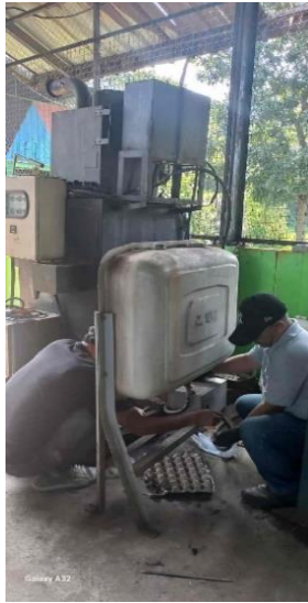
Figure 6. Disassembling of machines at PDU Cicabe, Bandung City
