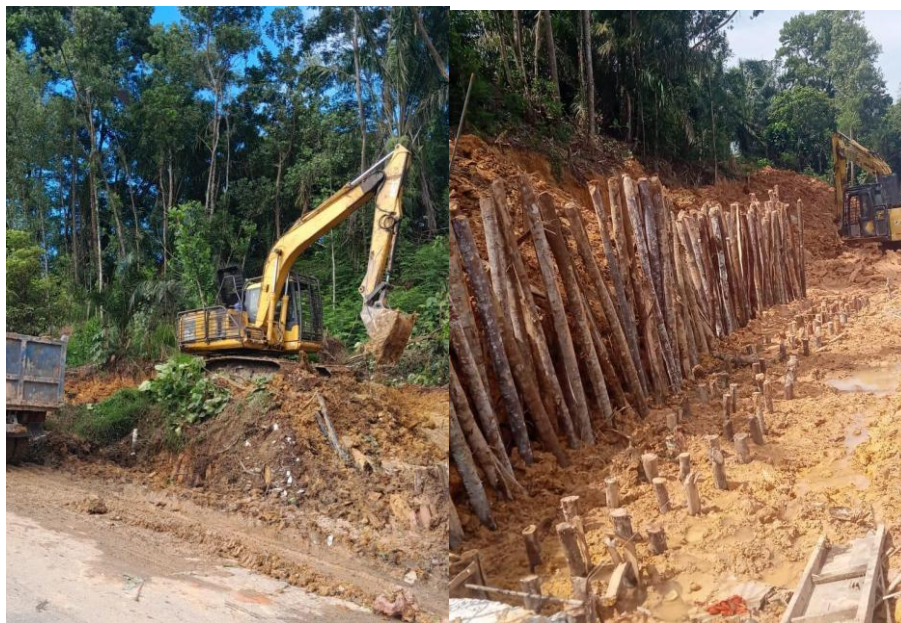
Figure 1. Excavation Works Beneath Slopes
