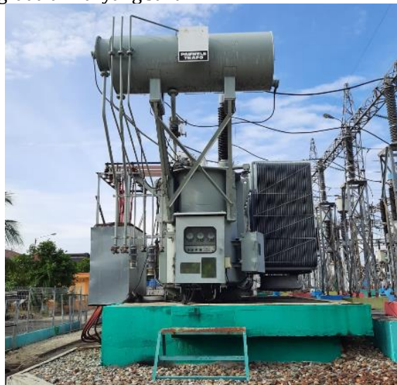
Gambar 1. Transformator Daya 2
